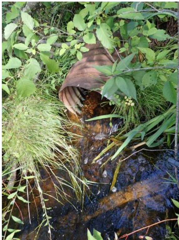
Figure 3.1.2-6. Corrugated steel pipe conveying Blackwater Creek Tributary 2 beneath a forestry road in Reach 2, approximately 1.25 km upstream from Normans Road.
