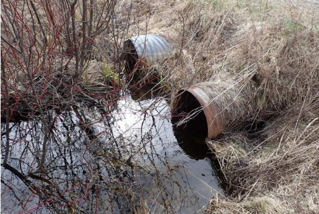
Figure 3.1.2-5. Corrugated steel pipes that convey Blackwater Creek Tributary 2 beneath Norman's Road. Most of the flow is conveyed by the culvert on the right.
