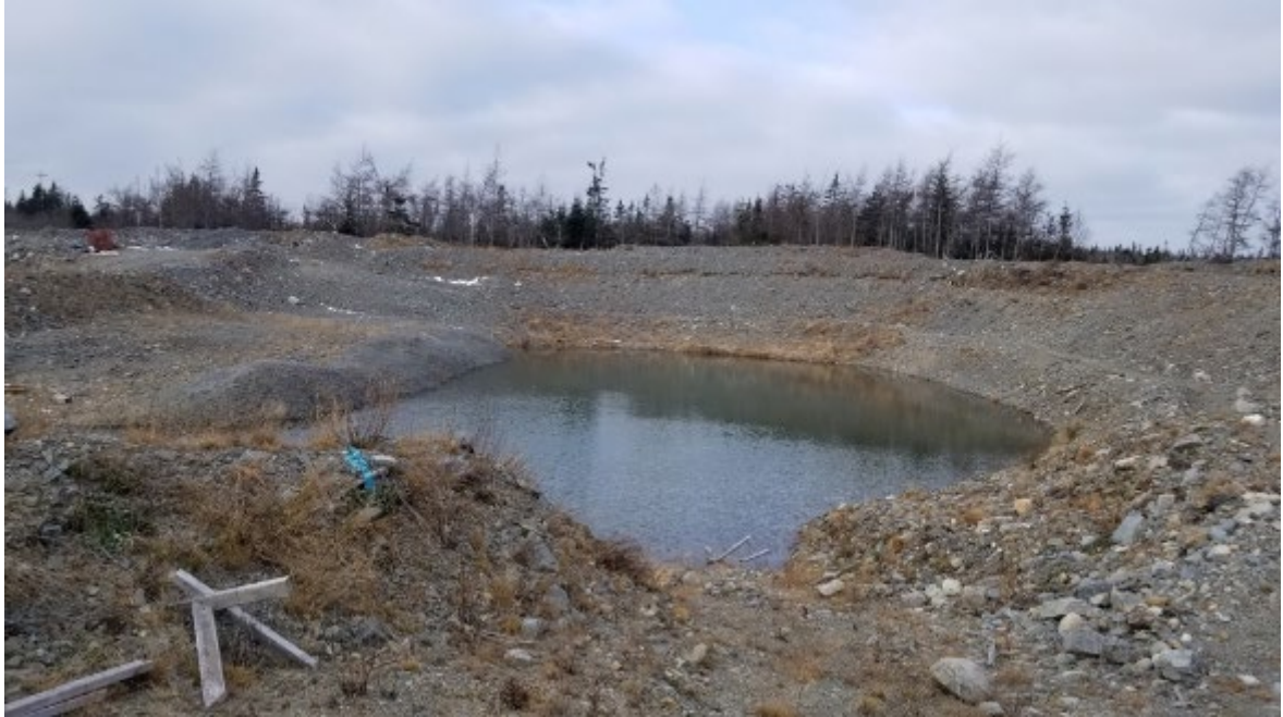
Figure 12-20: The flooded underground portal demonstrates the depth of overburden to bedrock
